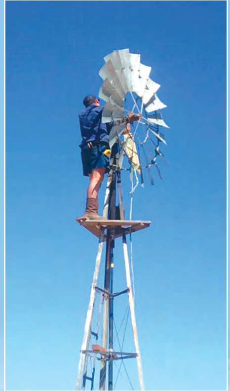
Shawn servicing the windmill head. ▲
